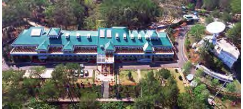
Aerial View of NE-SAC
