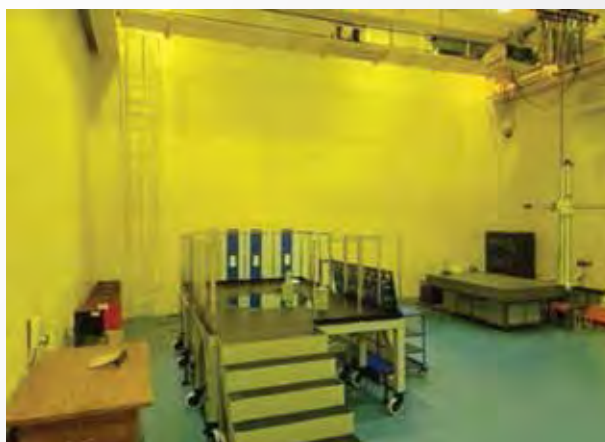
Clean Room for Gaganyaan CE20 Engine integration activities
