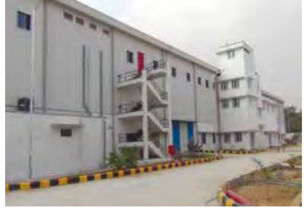
ICMF Main Hangar
